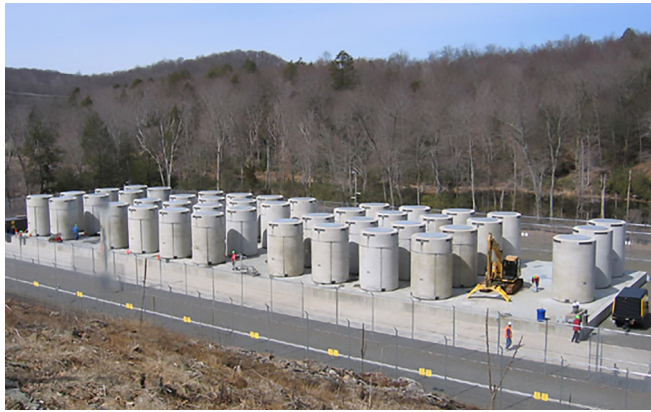
fig (6): Dry Casks Storage at the Connecticut Yankee Atomic Power Company [Source: Connecticut Yankee Atomic Power Company]
